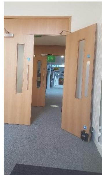
*Door fitted with a hold open device which releases in the event of a fire alarm*
