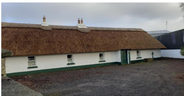
The Thatched House at Ballynagappagh, December 2020
